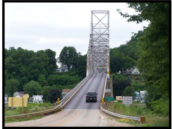
The Lansing Bridge crossing the main channel of the Mississippi River
